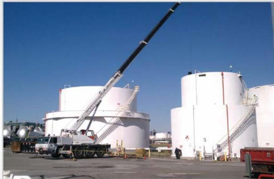
BP Terminal: Removal of the roof off the main product recovery storage tank to clean and perform the tank's 10 year inspection.
