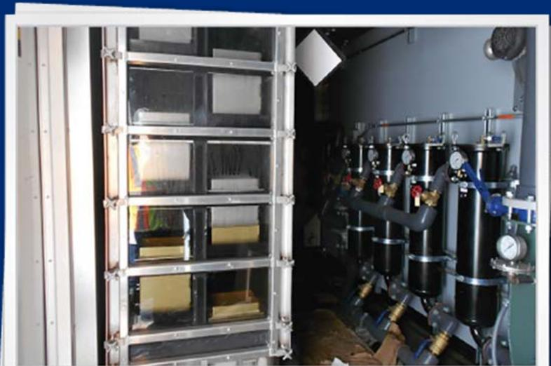
BP Terminal: Air stripper and bag filter units part of the BP groundwater treatment system.
